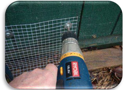
Attaching hardware cloth using a cordless drill/driver, lath screws and fender washers
