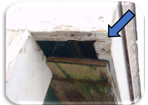
A missing piece of wood on the underside of this soffit makes it easy for birds or squirrels to enter
