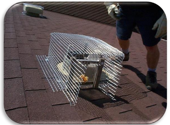
Wire-mesh installed over a repaired plumbing mat around a roof vent pipe. A raccoon had torn up the shingles and the plumbing mat to get into the attic. The mat is installed with lath screws and fender washers. The screws are daubed with waterproofing caulk. Note the "cap" of wire mesh on the pipe to exclude small birds and squirrels
