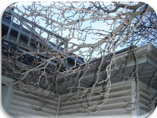
Branches close to the house make it easy for animals to get up to your roof, soffit, and chimney
