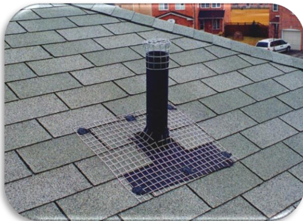
Wire-mesh installed over a repaired plumbing mat around a roof vent pipe. A raccoon had torn up the shingles and the plumbing mat to get into the attic. The mat is installed with lath screws and fender washers. The screws are daubed with waterproofing caulk. Note the "cap" of wire mesh on the pipe to exclude small birds and squirrels
