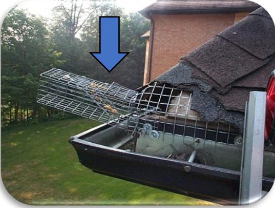
A one-way door (arrow) and exclusionary mesh installed on a squirrel entrance hole on a corner of a roof
